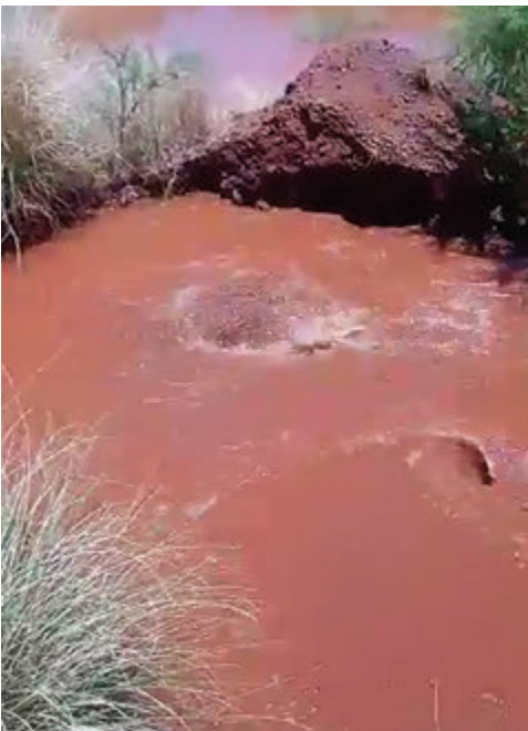
Water gushed from a burst pipe.
